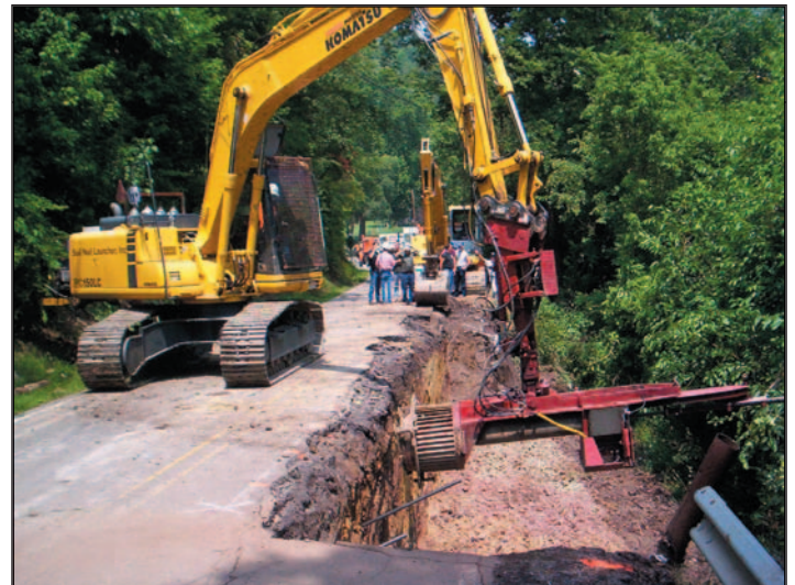
Above: Soil Nail Launcher used to stabilize rural road in Ohio
